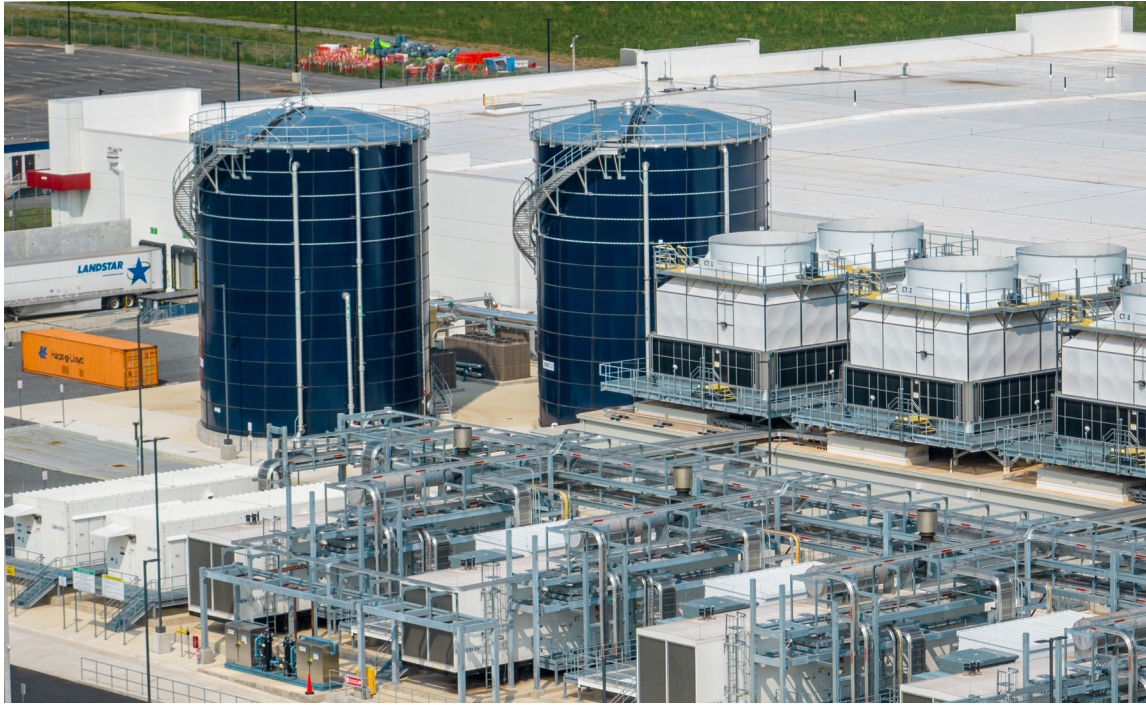
Infrastructure includes diesel generators, chillers and water storage tanks, Hugh Kenny, PEC.
